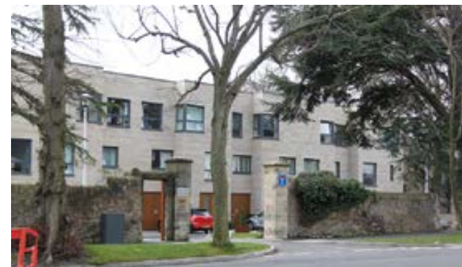
Boundary walls in villa areas—Newbattle Terrace Boundary walls are extremely important to the character and appearance of villa areas. The size and number of new openings to them should be minimised.
