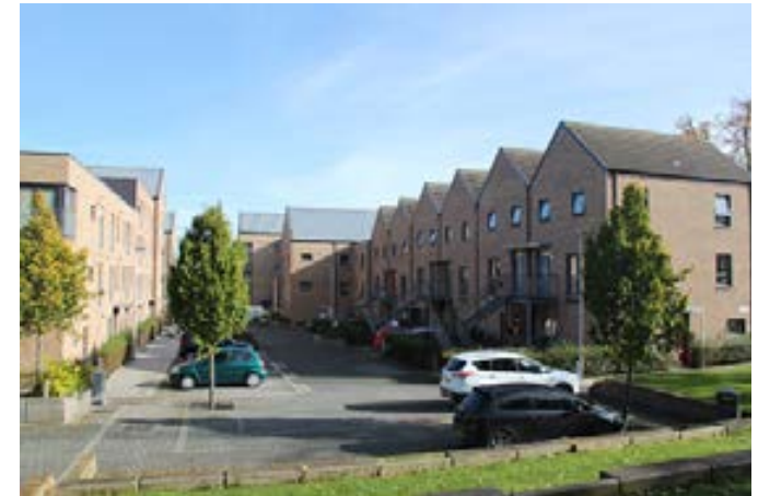
Minimising energy use through careful design—Garvald Street This housing development achieved a BREEAM excellence award in recognition of its high standards of sustainability. It achieves this through a range of measures including insulation, airtightness and heat recovery.
