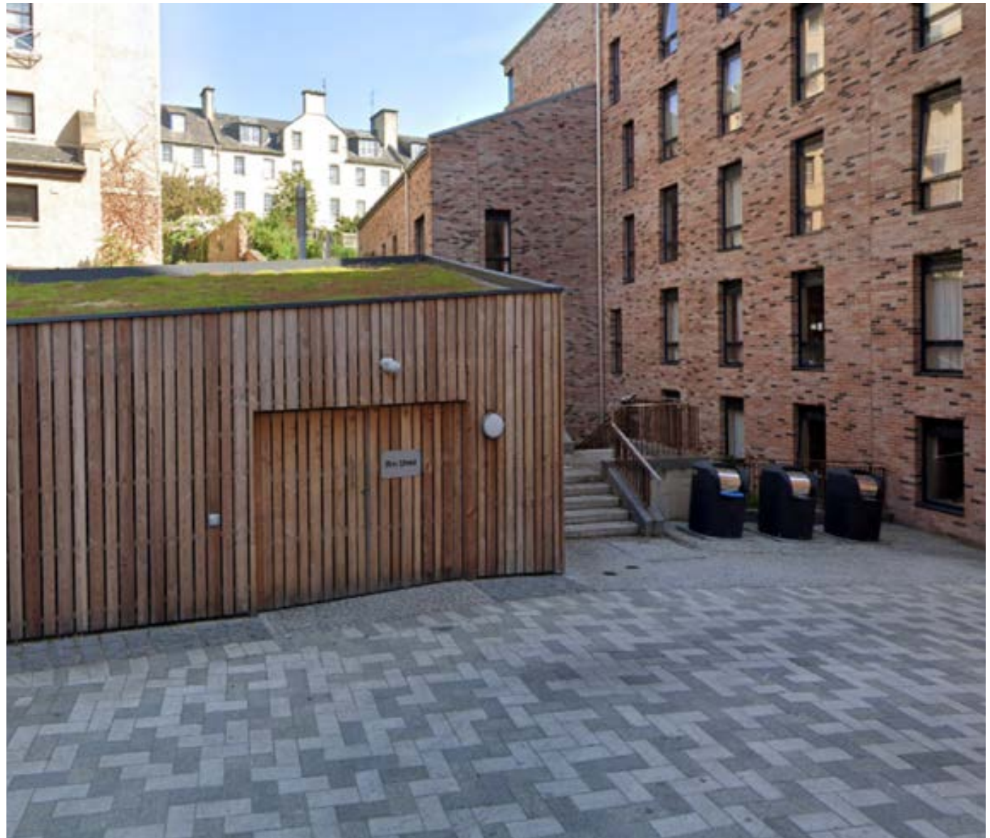
The use of bins with underground storage at Morgans Lane helps to minimise the impact of waste collection facilities.
