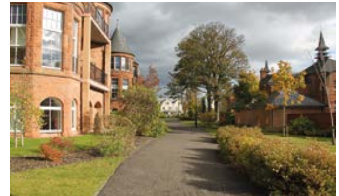
Former City Hospital - Greenbank
