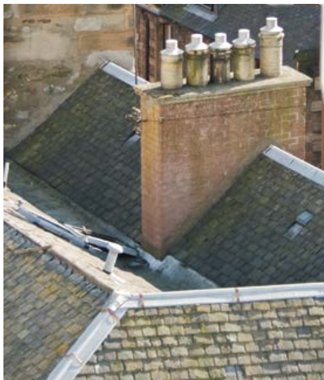
Traditional roofing materials Slate, Lead and zinc are traditional roofing materials used in Edinburgh—seen here from the Museum of Scotland's roof.
